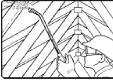
Treating Attic Areas
